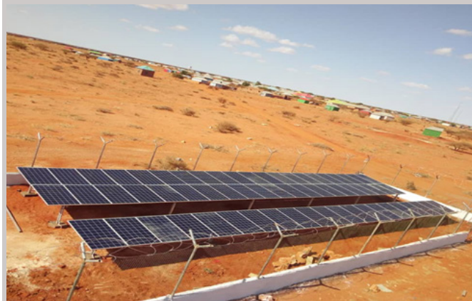
Solar panels have been installed in Galmudug
